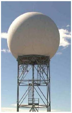
The Weather Surveillance Radar, 1988 Doppler (WSR-88D), also known as NEXRAD, is the most advanced operational weather radar in the world. The fleet of 159 WSR-88D radars operate 24/7 to support the weather warning and forecast missions of the National Weather Service, FAA and DoD. Additionally, realtime radar data is made available to the nation's academic and commercial weather enterprise.
